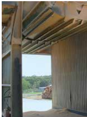
View into a hopper from below. With large-grained bulk goods, which may cause serious localised wear, lining the exposed parts with Matrox will considerably prolong the life span of the hopper.
