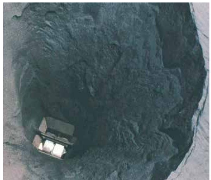
Rathole: The centre portion of the bin empties first in the form of a funnel (Photo Courtesy of Solids Handling Technologies, Inc.).
